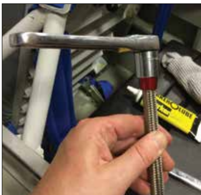
Using a socket to help install the hose end fitting.
