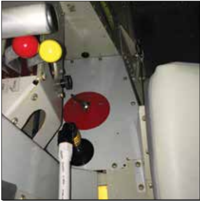
Fuel hose connection at the fuel selector.
