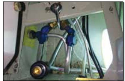
Fabricated fuel line correctly oriented and installed.
