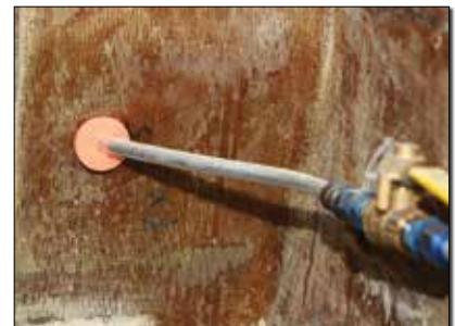
Some soapy water helps to fit the grommet in the bulkhead opening.
