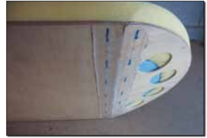
Angled backing frames should be reinforced with fiberglass.
