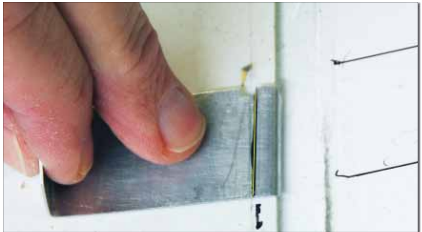
Now transfer the mark to the cowl. Repeat to create a dotted cutting line, and you'll get a conformal line between the cowl and the fuselage.
